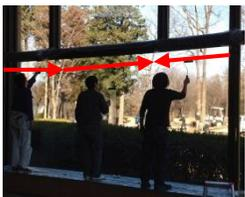
Apply vertically from the top on both sides to the center with little pressure. (30%)
