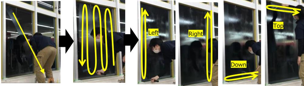
① Put the required amount of liquid (25 g / m<sup>2</sup>) in the tray and let it suck into the special roller.
