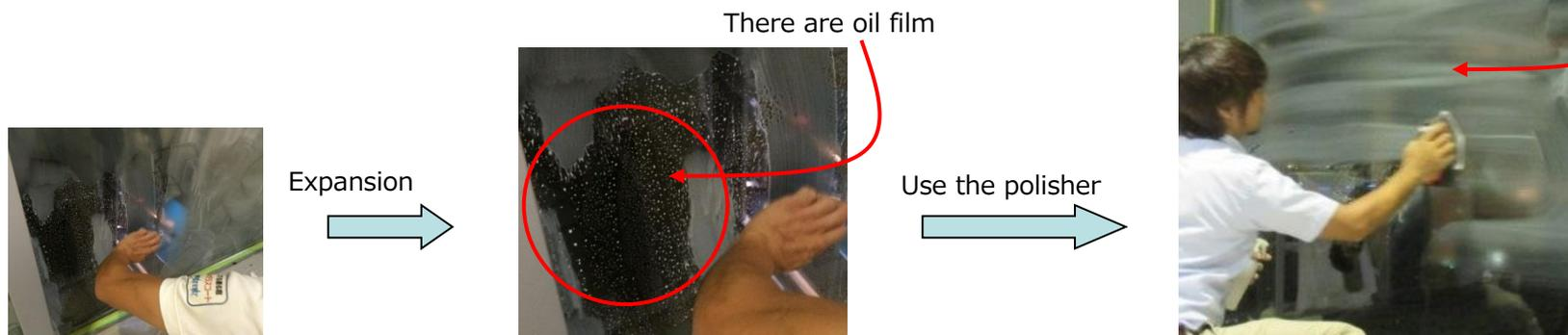
When there are many parts of oil film, it is better to use the polisher machine to polish the glass.
