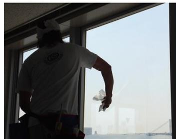
1) Put 5 ~ 10g / m<sup>2</sup> of glass cleaner to buff and polish while spraying the water to spread on the entire glass. Polish until the glass becomes hydrophilic state (do not repel the water).
